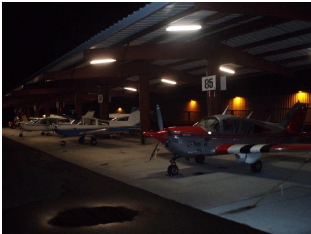
Figure 74 – Example of linear fluorescent lighting under the shades. These fixtures are unshielded, largely outside of the amber light spectrum, and could benefit from occupancy controls. The LPS lights seen in the background are part of the hangar lighting.
