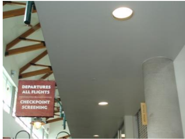
Figure 25 – Recessed can lighting in the lobby.
