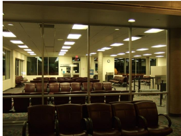
Figure 27 – Linear fluorescent T8 lighting in the drop ceiling in the security area.
