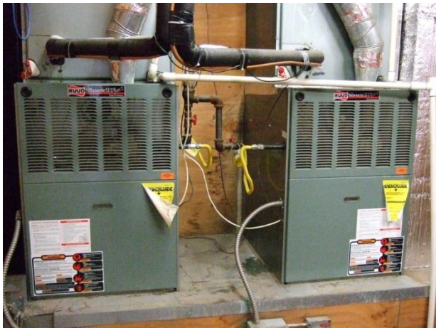
Figure 16 – Example of two furnace units.
