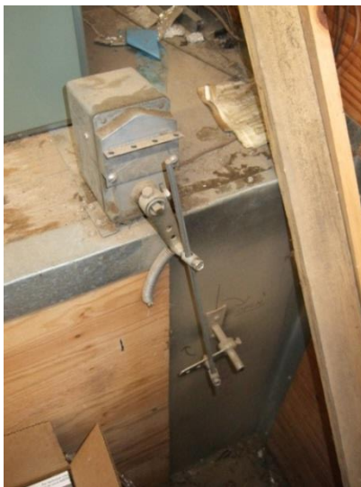
Figure 65 – Outside air damper and controls.
