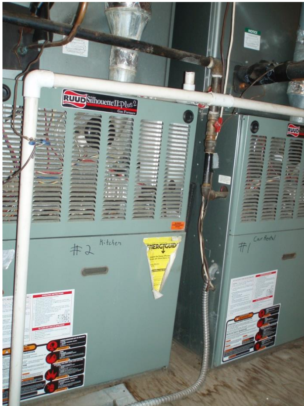
Figure 95 – The furnaces serving the kitchen and car rental areas share a common return plenum box.
