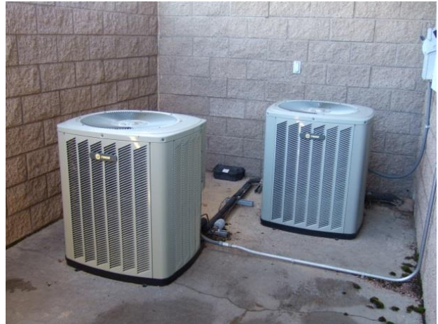
Figure 36 – The condenser units on grade next to garage bays.
