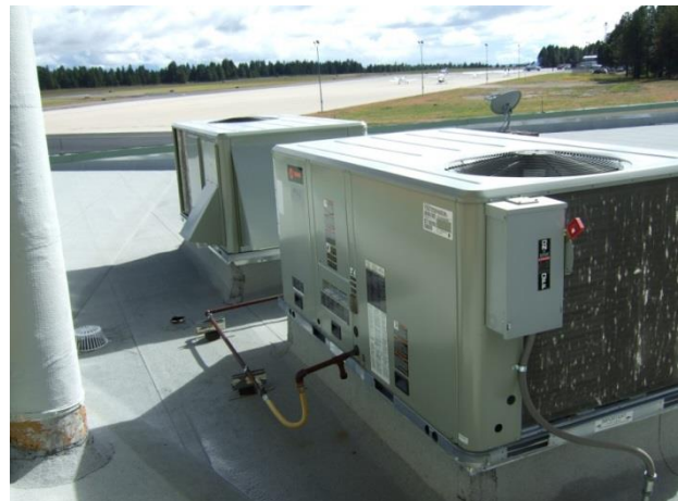
Figure 17 – RTU-1 and RTU-2 serving the security area.
