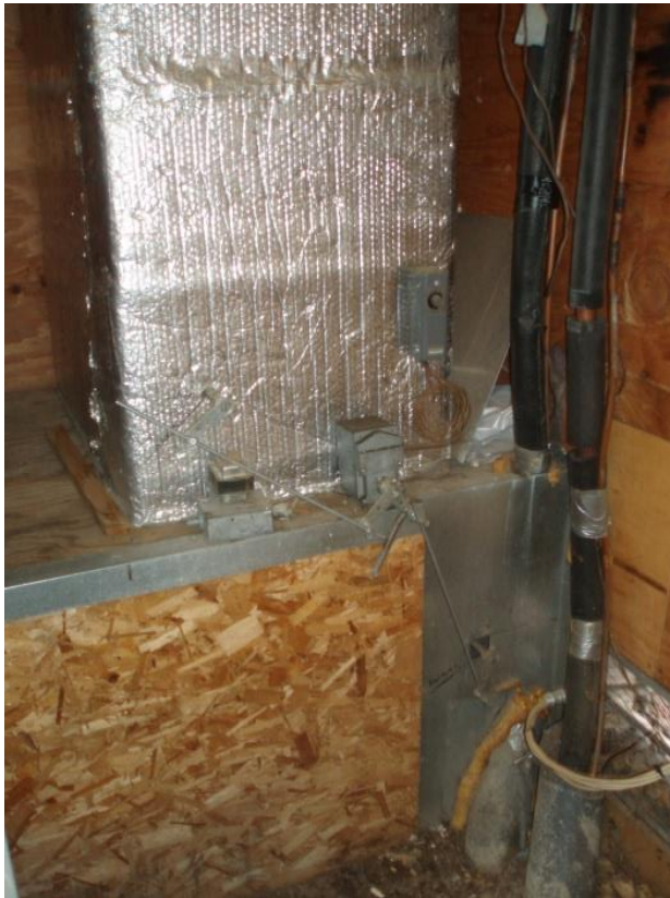
Figure 18 – Example furnaces with return plenum box and outside air damper.
