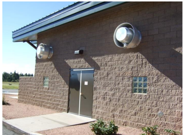
Figure 40 – Apparatus/equipment bay exhaust fans.
