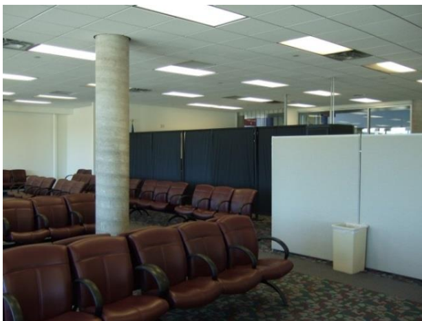
Figure 58 – T8 fixtures located in the security area.
