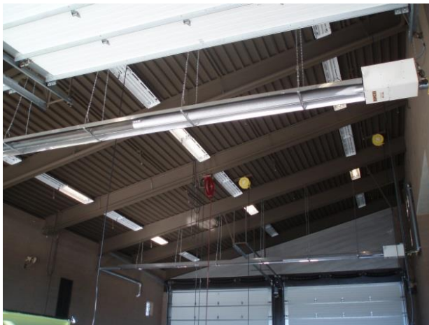
Figure 61 – The linear fluorescent lights that are on in this photo are a good candidate for relamping with linear LED.
