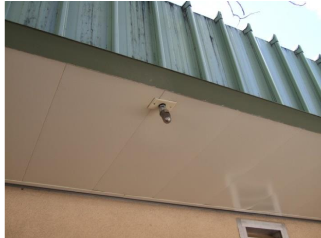
Figure 33 – Photocell sensor for parking lot lighting.
