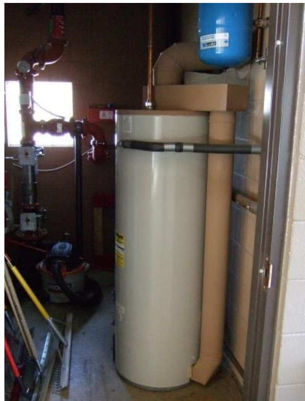
Figure 42 – Laundry and garage wash basin water heater.
