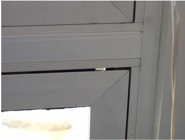
Figure 12 – Example of air gap in window frames in the administrative area.
