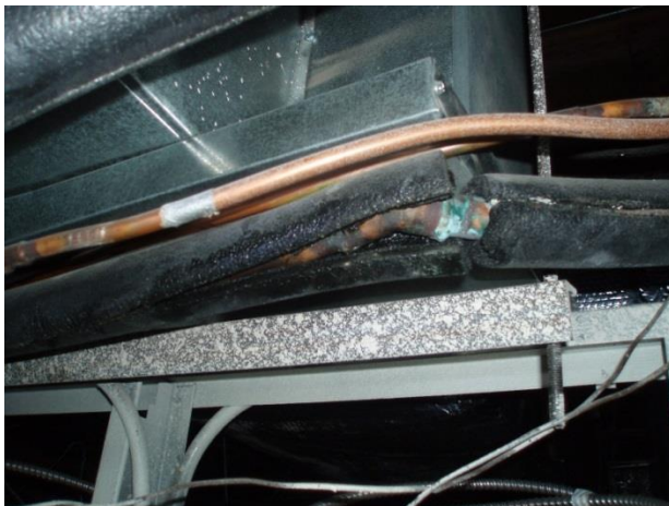
Figure 82 – Refrigerant pipe insulation that is damaged above the administrative area. This is resulting in condensation dripping onto the ceiling tiles below.
