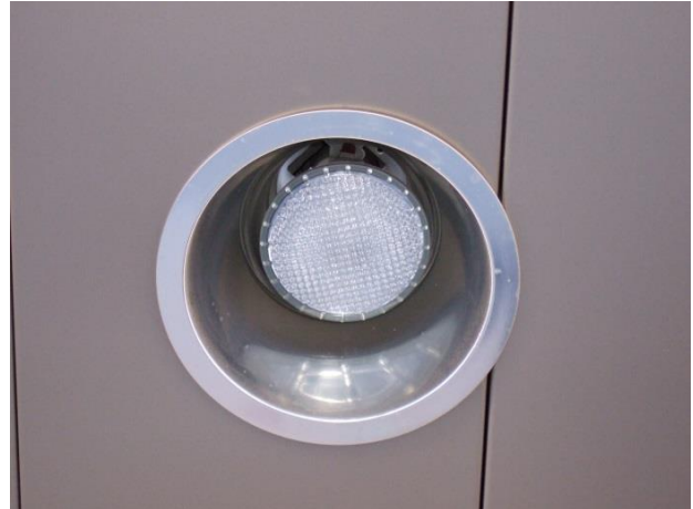
Figure 48 – Exterior recessed canned light with a halogen lamp.
