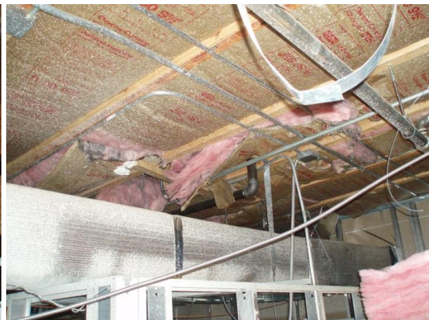
Figure 11 – Typical roof insulation detail in areas of the building with a flat roof.
