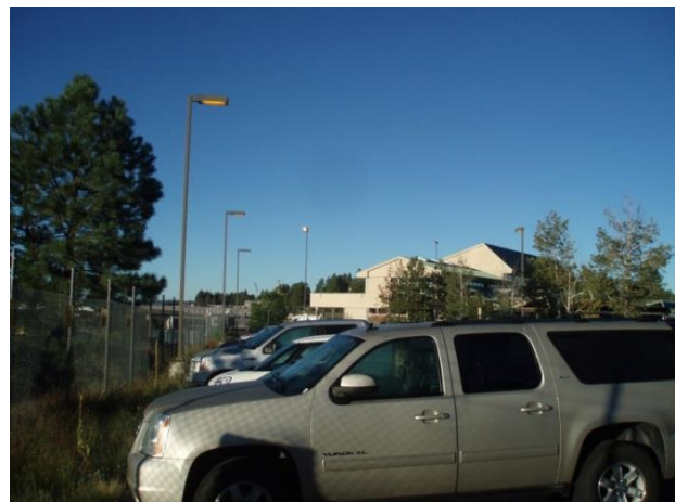
Figure 70 – Parking lot lights remain on late in the morning due to the photocell location.
