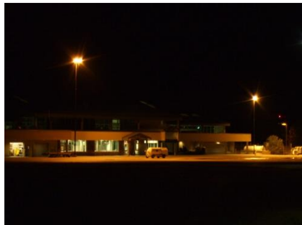
Figure 76 – The Main Terminal apron is lit with high pressure sodium flood lamps.
