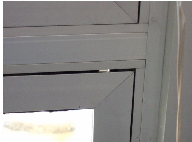
Figure 90 – Daylight can be seen through gaps between the window and frame, resulting in air leakage.
