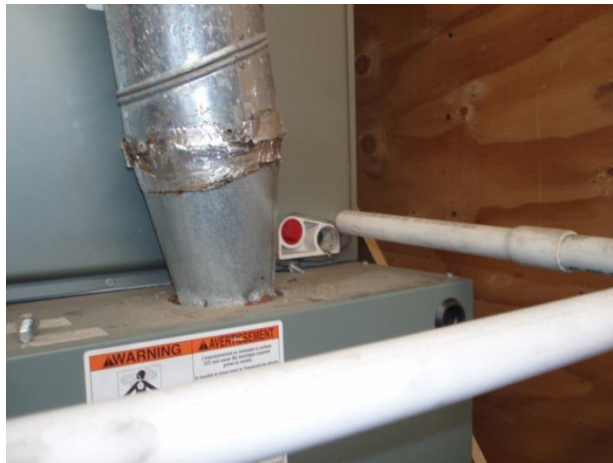
Figure 83 – The cooling coil condensate pipe is disconnected from furnace F-9.
