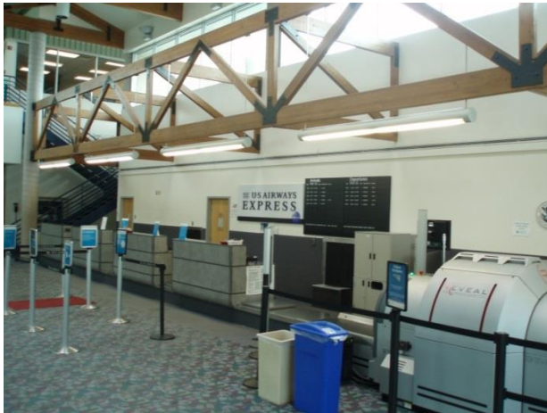
Figure 26 – Linear fluorescent T8 lighting in the ticketing area.
