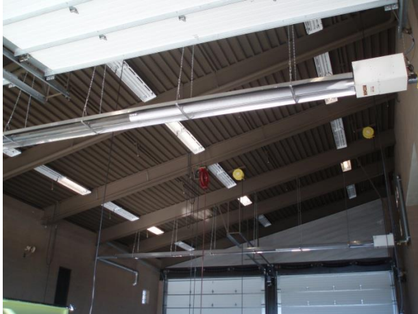
Figure 43 – High bay fluorescent lighting in the apparatus bay. Some lights stay on for emergency lighting.
