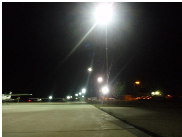
Figure 75 – The GA/FBO apron is lit with pole fixtures with metal halide lamps.
