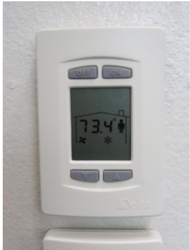
Figure 19 – The typical programmable thermostats for furnace and rooftop unit control.
