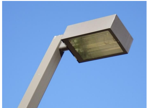
Figure 50 – A fully shielded LPS pole mounted fixture.
