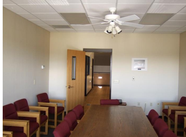
Figure 44 – Linear fluorescent lighting with fan ceiling fixture lighting in the office spaces.
