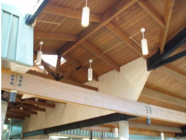
Figure 28 – An example of pendant can lights in the entrance canopies.
