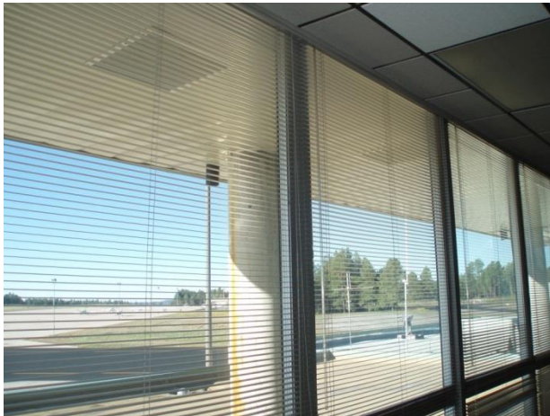
Figure 89 – 2 nd floor conference windows with single panes and storm window coverings.
