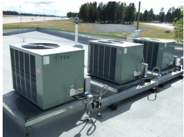
Figure 21 – The typical rooftop condensers serving the furnaces.
