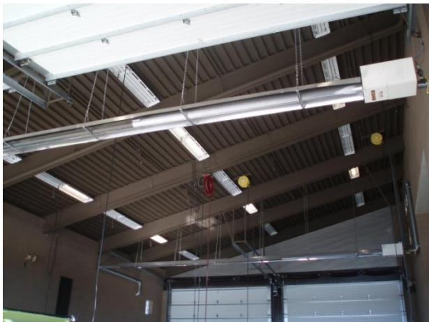
Figure 39 – Radiant heaters in apparatus/equipment bays.
