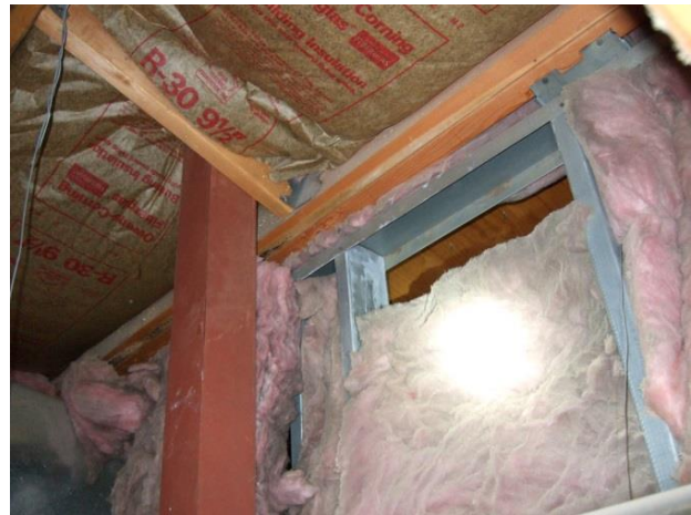
Figure 92 – An example of failing insulation below the roof, allowing cold air to circumvent the thermal barrier. The steel stud wall cavity seen here insulates the space above the ceiling from the space in the overhang.
