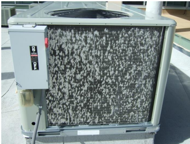
Figure 81 – An example of weather/hail damage on rooftop condensing units.
