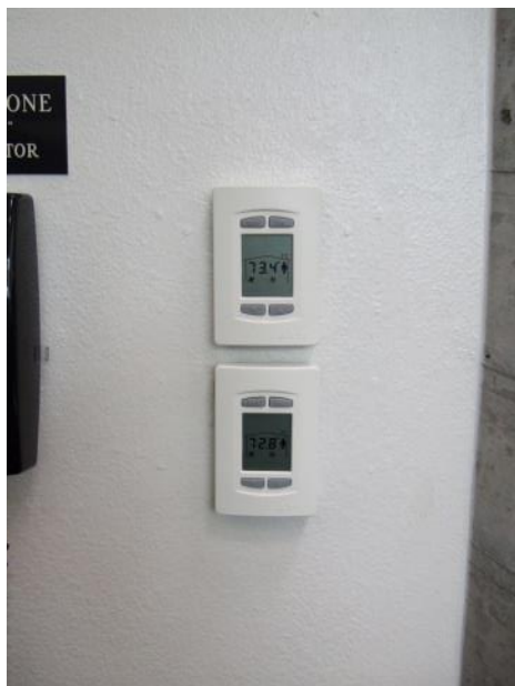
Figure 52 – An example of thermostats in close proximity to each other.
