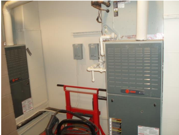
Figure 35 – Typical furnaces serving the ARFF living quarters area.
