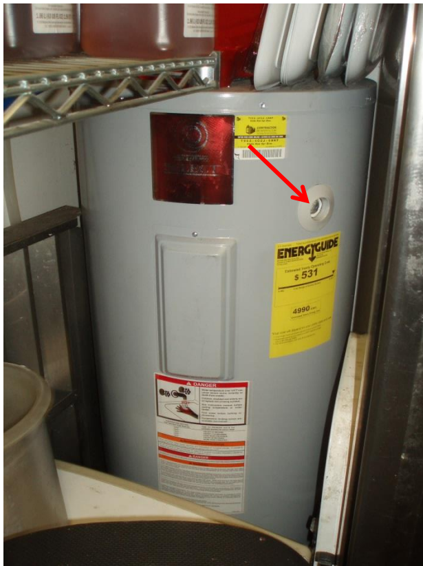
Figure 88 – The water heater serving the kitchen is without its T&P valve.
