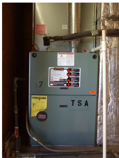
Figure 66 – A standard efficiency existing furnace.
