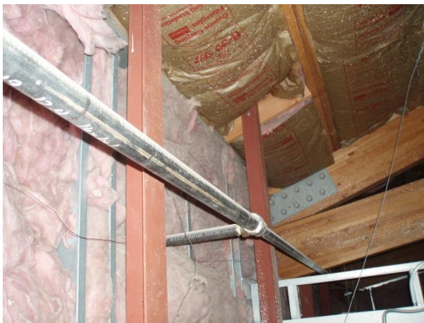
Figure 10 – Typical wall-to-roof insulation detail in areas of the building with a pitched roof.
