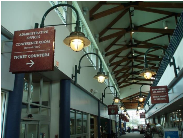
Figure 24 – A variety of lighting types serve the main terminal lobby, including the street lamps and pendant can lights.
