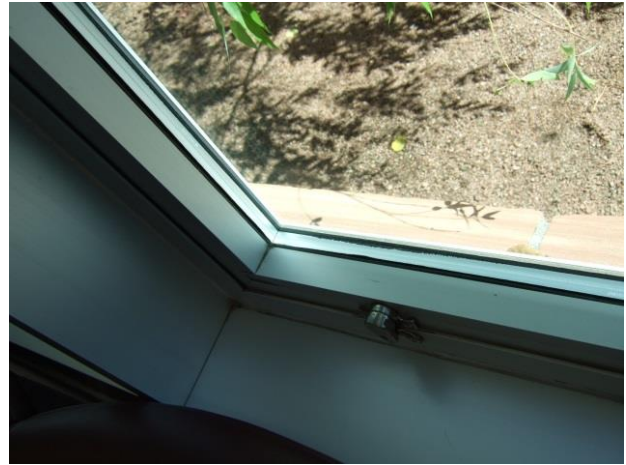
Figure 13 – Double pane window typical throughout the non-administrative areas of the Terminal.
