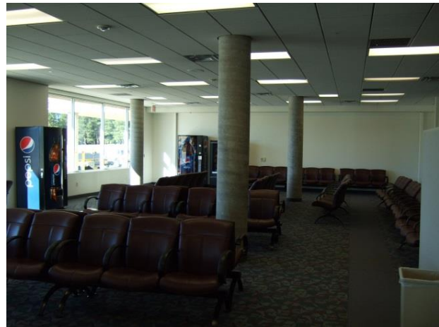
Figure 54 – Security area lights near the windows are candidates for daylighting controls, but this was determined to be less cost effective than occupancy controls.
