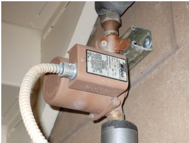
Figure 68 – The current domestic hot water recirculation pump.
