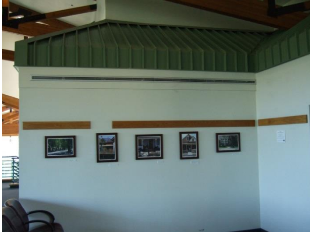
Figure 78 – An example of a linear supply air diffuser in 2nd floor lobby (the aluminum register located near the top of the wall and just below the decorative metal roof). No air could be felt moving from these diffusers.
