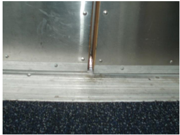
Figure 80 – Gaps resulting in air leakage were observed on exterior doors, such as this one leading to the apron.
