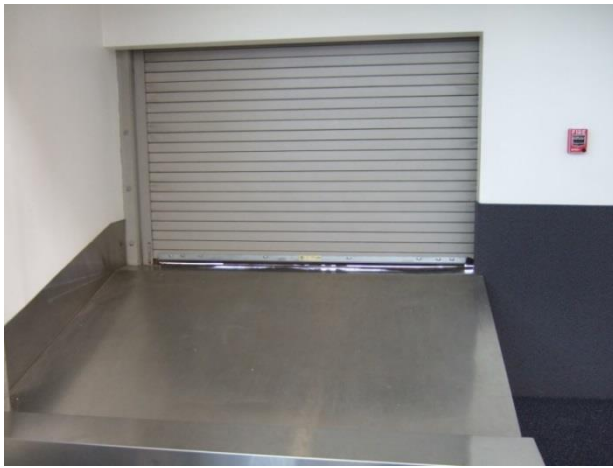
Figure 79 – Baggage claim door with air leaks around the perimeter.
