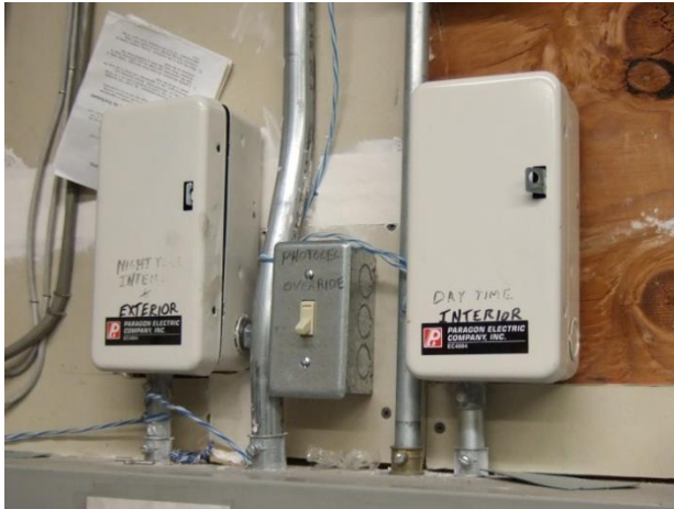
Figure 32 – Lighting timers and controls for interior and exterior lights.
