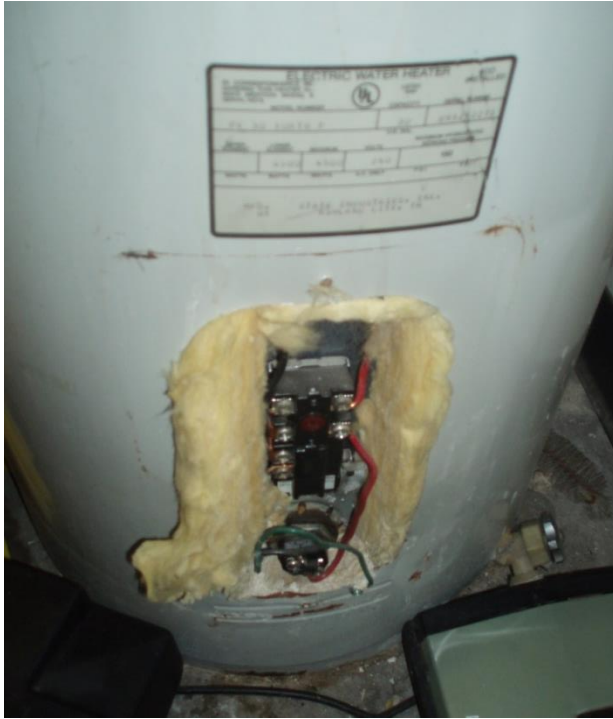
Figure 87 – The main lobby restrooms water heater with exposed heating element electrical terminals.
