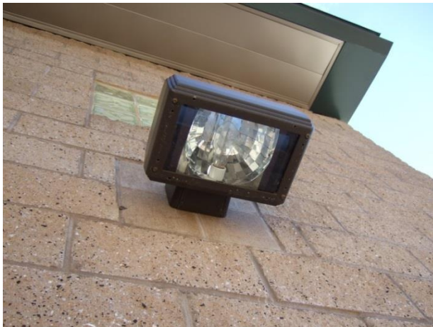
Figure 49 – A fully shielded LPS wall pack fixture.
