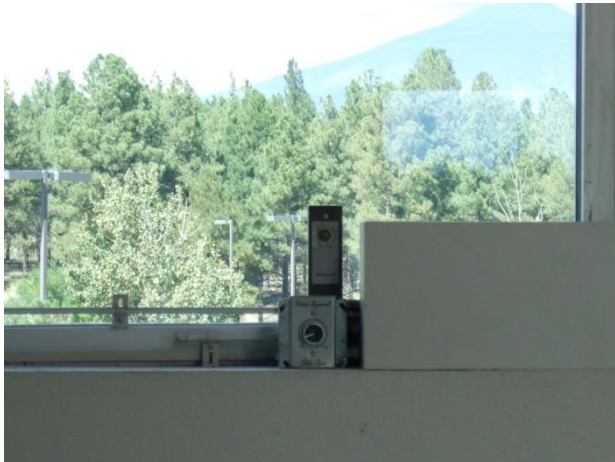
Figure 14 – Automatic window controls on the upper windows in the atrium that have been abandoned.
