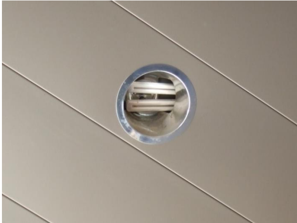
Figure 47 – Exterior recessed canned light with compact fluorescent lamps.
