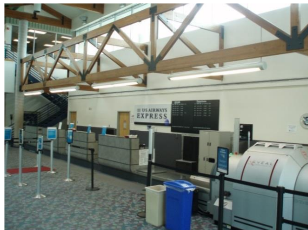
Figure 59 – T8 fixtures located at the ticketing and TSA areas.
