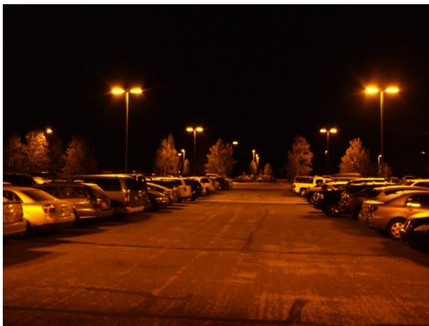
Figure 77 – Pole mounted LPS lamps in the Terminal parking lot.
