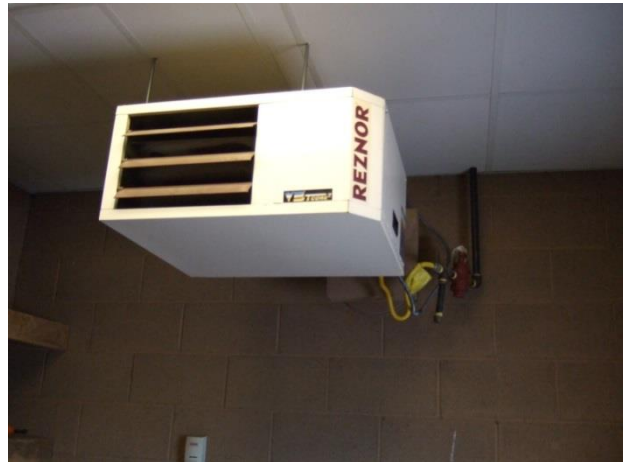
Figure 38 – Gas unit heater serving the garage shop space.
