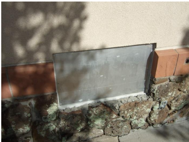
Figure 20 – An example of an outside air intake for a return plenum box that has been blanked off.
