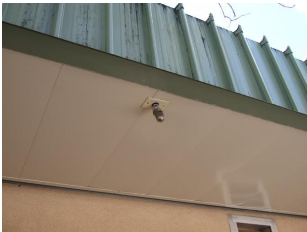
Figure 69 – The current photocell location under an overhang.
